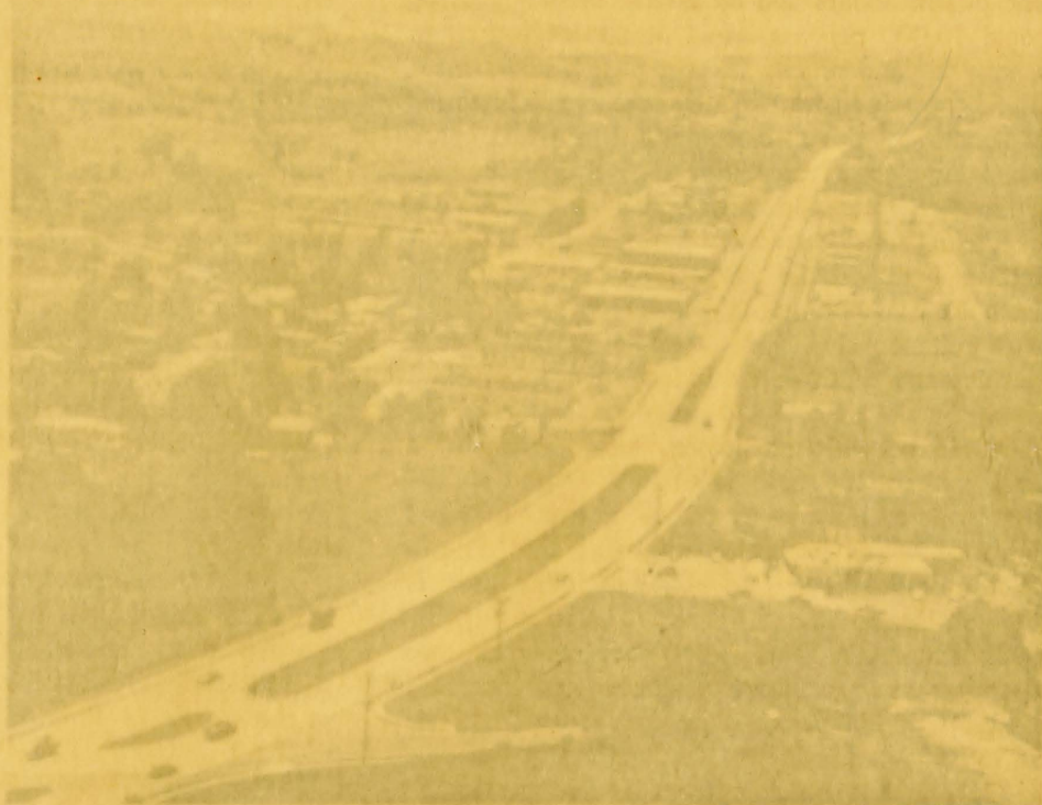
With an area of 3,500 square miles, Puerto Rico has some 1,000 miles of modern hard-surface roads. (USISI)
