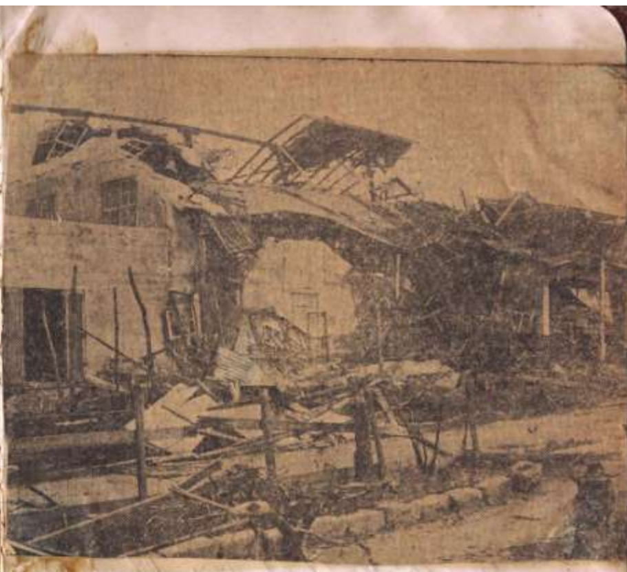
A factory that was destroyed by the storm.
