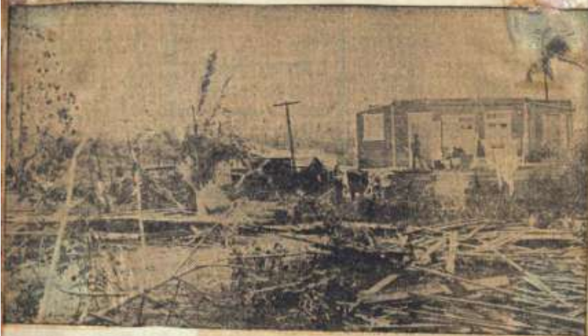
A town destroyed by the hurricane
