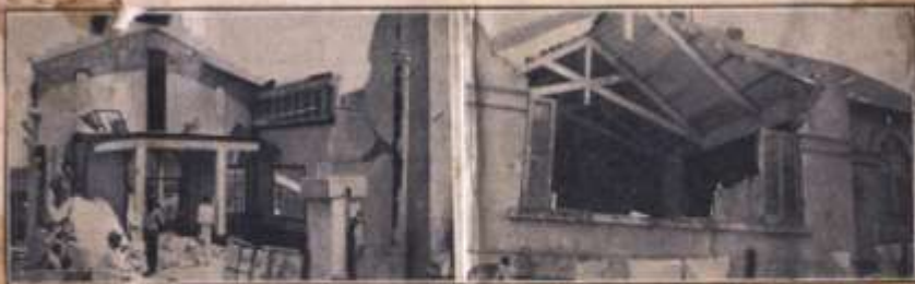
These are low masonry houses destroyed by the storm. In Yabucoa
